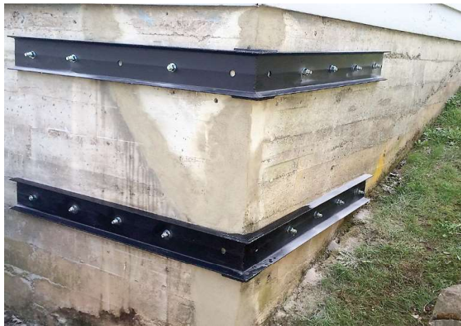
CUSTOM STEEL C-CHANNEL BRACE
