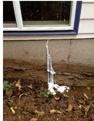
CRACK INJECTION
