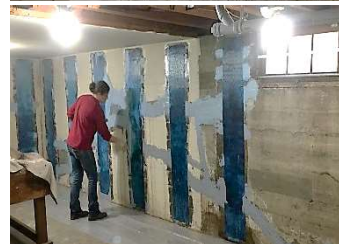
CARBON FIBER REPAIR AND STRENGTHENING
