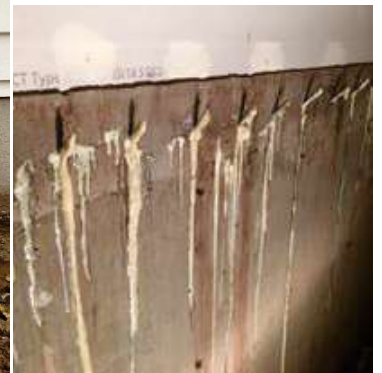
CRACK INJECTION
