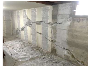
CRACK INJECTION
