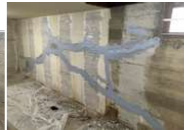
CRACK INJECTION
