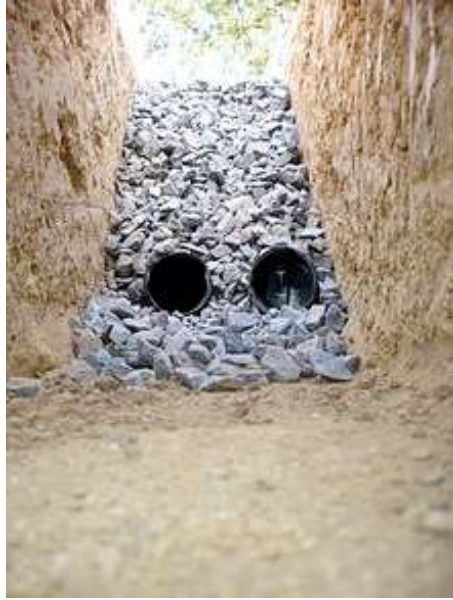
Exterior french drains
