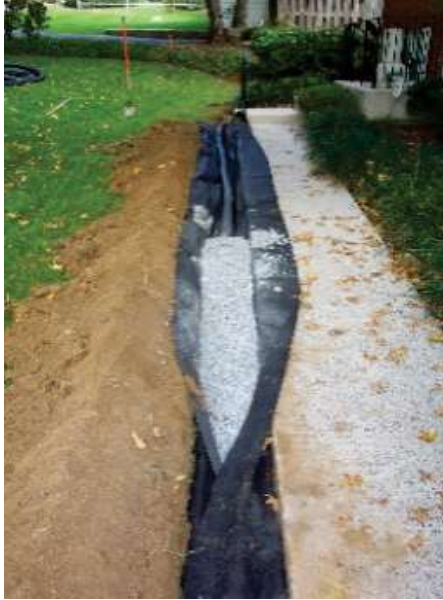
Exterior french drains
